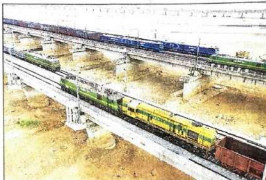
An aerial view of the trial run of trains on Dehri-Sonengar-rail bridge
